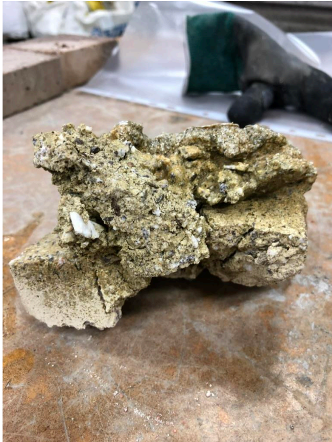
Figure 28 Melted concrete sample
